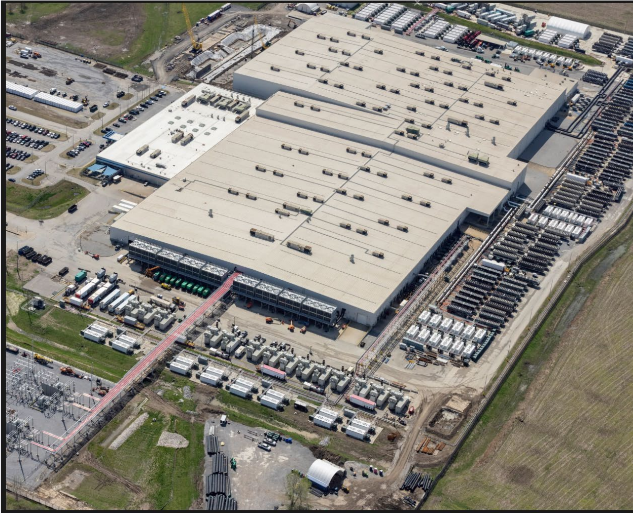
The xAI datacenter in Memphis. Photograph: Steve Jones/Flight by Southwings for Southern Environmental Law Center
