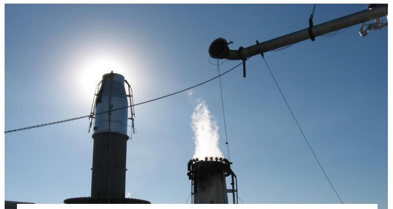
Low DRE. The lack of a visible flame and excessive steam at the flare tip are good visual indicators the flare is being operated at low DRE.
