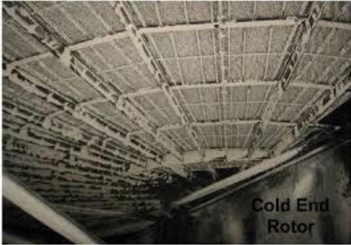
Rotary Air Preheater
