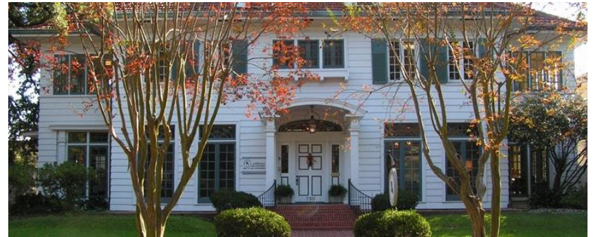
LMOGA House – 730 North Boulevard
